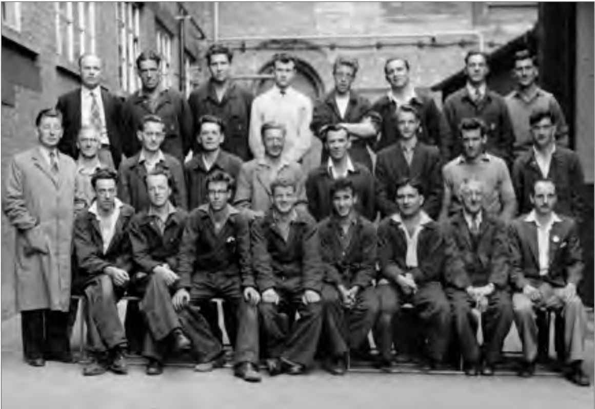
York Street, Belfast: PM Walker Team erecting air conditioning plant at Gallahers July 1960.
