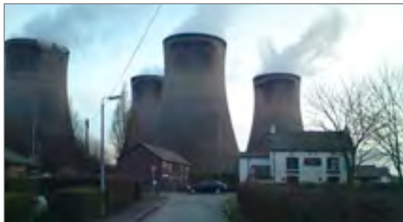
Cuerdley: In 1861 and 1871, James Ainscough (b 1832, Churchtown) and Alice Cookson (b 1830 Southport) lived at Moss Lane near Cuerdley Hall. What was pleasant low lying pastoral land was obliterated by the construction of the coal fired Fiddlers Ferry Power Station in 1961. 2010.
