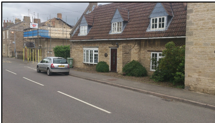
No 8 Bridge Street in 2015, the site of The Indian Queen
